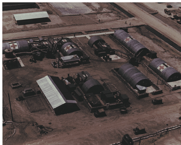
Figure 5-11. Aerial view of US Army MUST hospital facility in Vietnam. Reproduced from National Archives and Records Administration, record group unknown.
